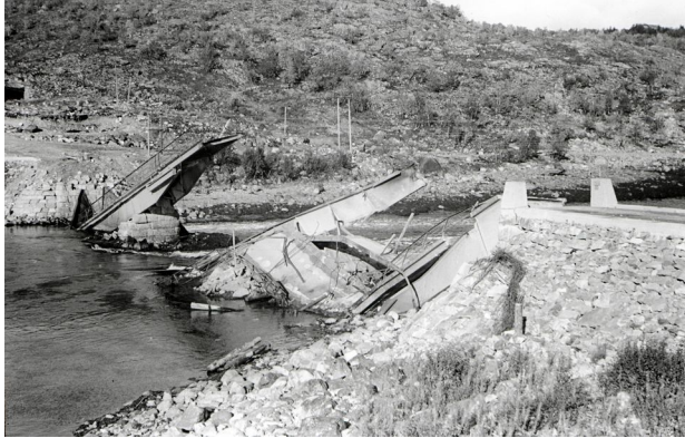
Strømmen Bridge was blown up by German forces as they retreated from Petsamo during “Operation Northern Lights” in 1944. Photo: Unknown photographer/Norsk vegmuseum, Statens vegvesen
